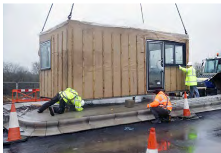
Locate onto capped-off services
