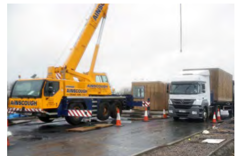
Second + third modules arrive by lorry
