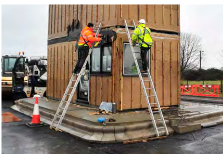
Weatherproof between modules
