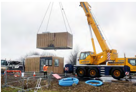
Repeat lifting operations
