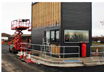
Clad in timber weatherboarding
