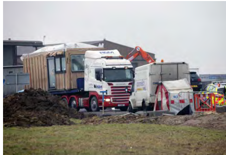
Prefabricated modules delivered by lorry
