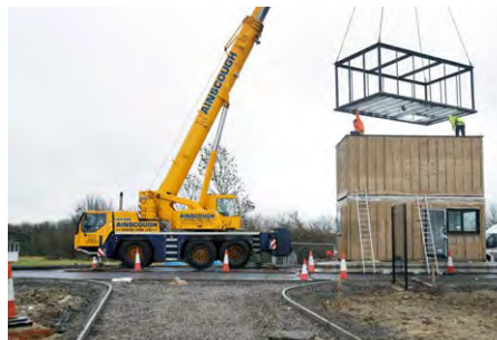
Crane lift of light-box module
