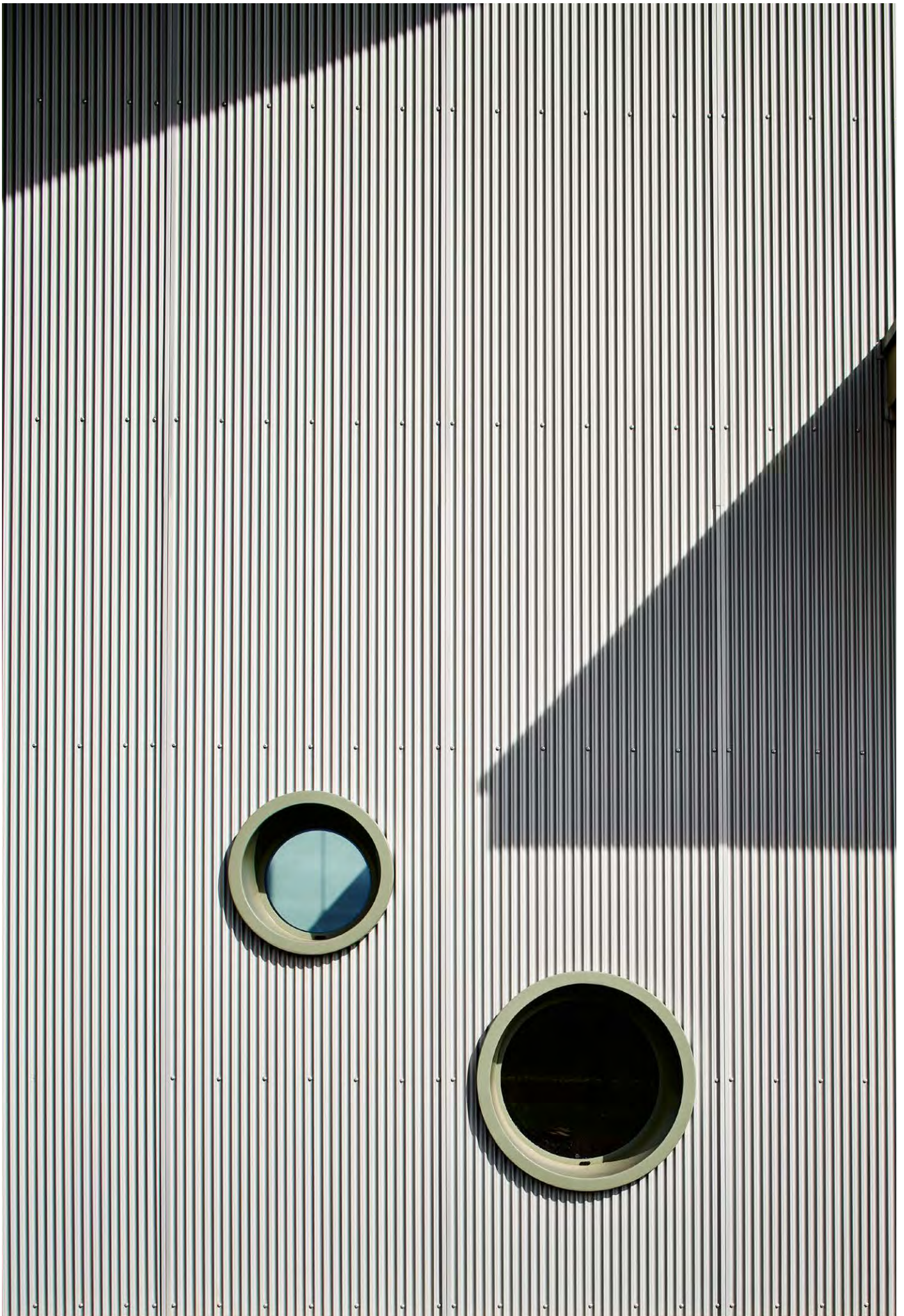
View of External sinusoidal metal cladding
