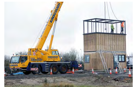
Fix light-box module to solid module
