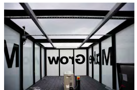
Fit-out and install lightbox glazing + signage
